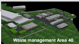
Waste management Area 40
