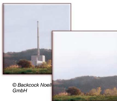
Removed NPP Niederaichbach
